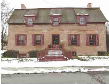
HISTORIC APPEARANCE - BRICK
