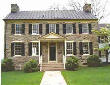
HISTORIC APPEARANCE - STONE
